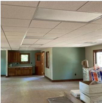
New staff office area
