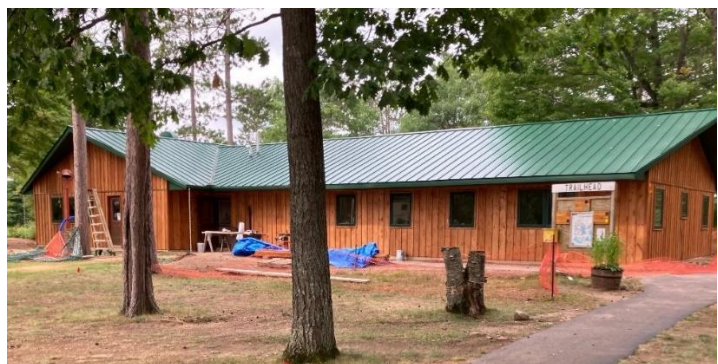
Front view of renovated Lodge with new siding
