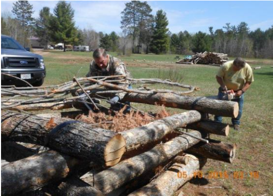
John Schulta and Tom Kramer are shown stuffing brush into the cribs.
